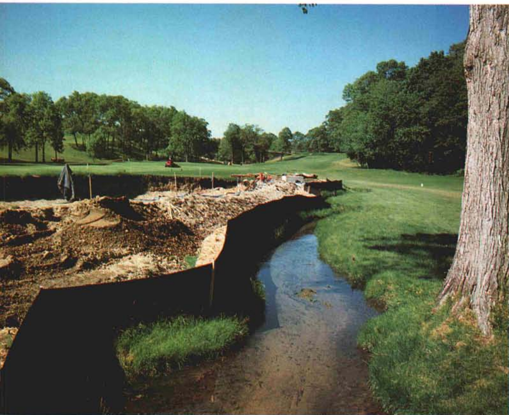
Pond construction at Brae Burn included protection of a nearby stream.
